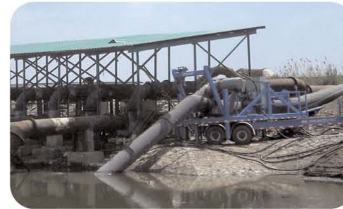
30" Mobile pump bypassing permanent pumps.
