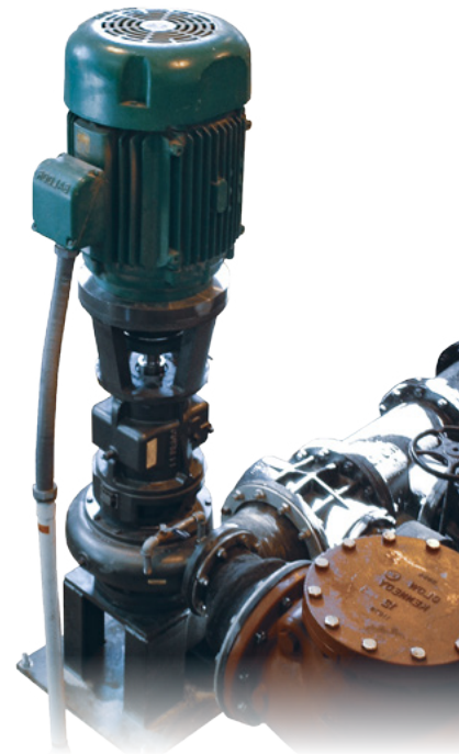
Chopper pump operating at a treatment plant.
